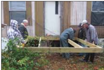
MOMC members build a deck in Tennessee.
