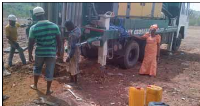
Drilling for water.
