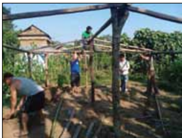
Building new homes
