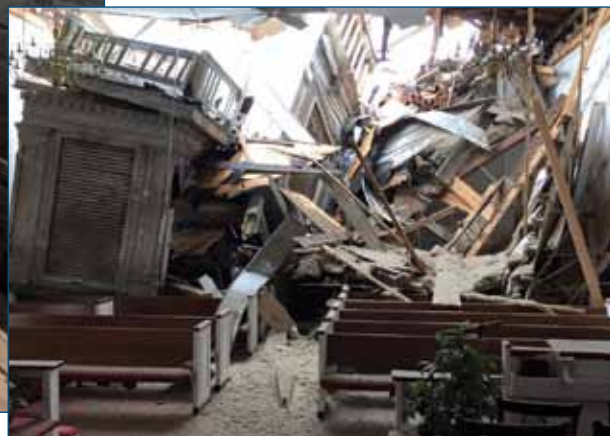
The steeple of First Congregational Church of Portland, Mich., became the church's most prominent pew-sitter as a result of the June 22, 2015 tornado that destroyed Portland's three historic hilltop churches and another storefront church.
