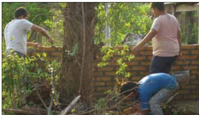
A new brick wall was part of the renovation project.
