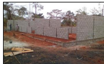
Building the foundation
