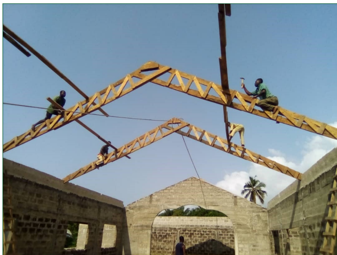
Word Alive Mission: Building the Ekpu church roof
