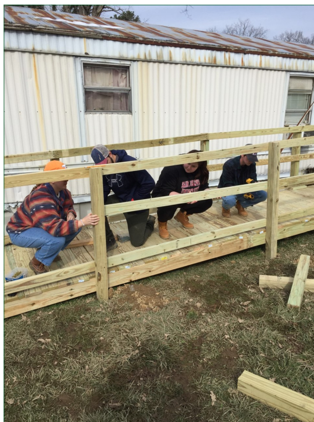
Building a wheelchair ramp
