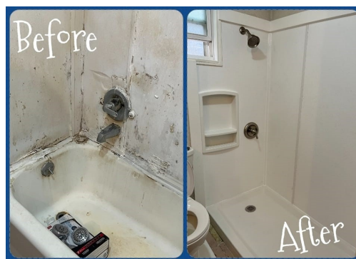
Home repairs for families in need
