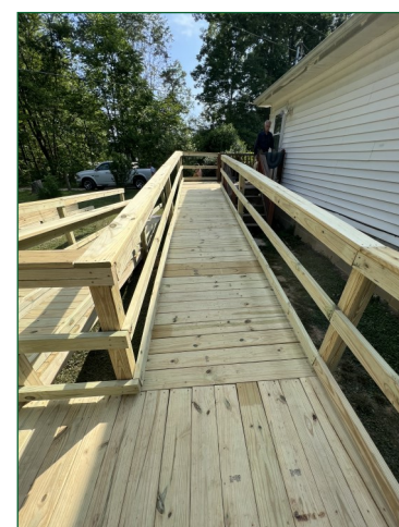
Newly constructed ramp at Morgan Scott Project
